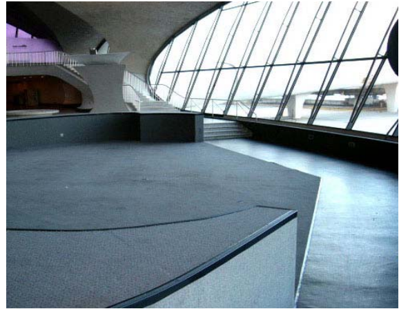
Sunken waiting lounge, Terminal 5 site
